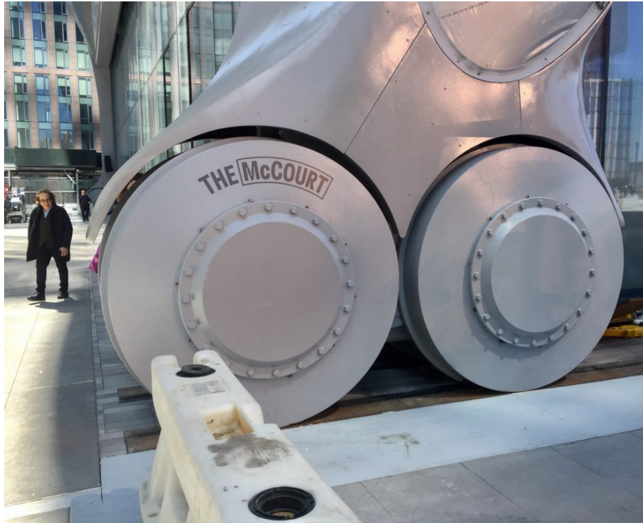
The wheels of The Shed's telescoping shell. Image courtesy Ben Davis.
